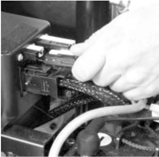
FIGURE 20. UNPLUGGING THE BATTERY HARNESSES
