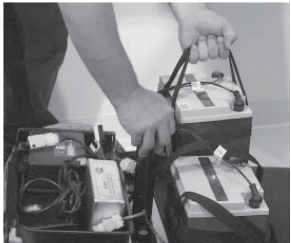
Figure 20. Lifting the Batteries
