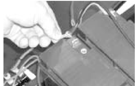
FIGURE 12. BATTERY CABLE REMOVAL
